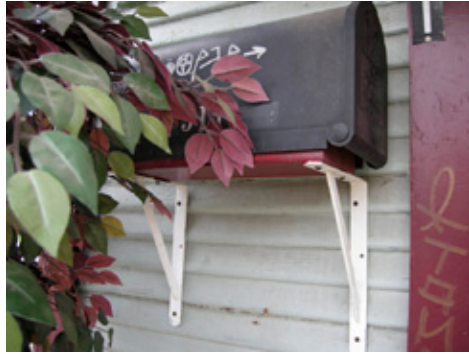
Brackets and a wooden shelf have been used to support this mailbox. The shelf was measured and cut and quickly painted to match the door frame. This mailbox scenario is a functional yet strange assemblage of efforts.
