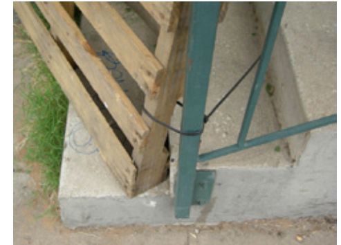
A pallet fastened to an iron handrail with a nylon zip tie becomes a quick and temporary blockade for a stairwell.
