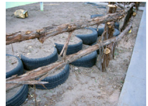
A sloping yard is leveled with stacked tires. Collection and placement of the tires required foresight and preparation. Though filled with dirt, they are otherwise unaltered. The tires are literally embedded into the environment and will provide long-term erosion prevention.
